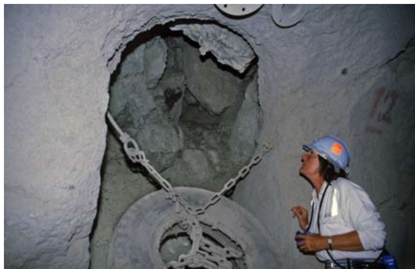
Fig. 7. Looking through a drawpoint in a scraper drift at the 860-m level in the Bultfontein mine. Beyond the concrete arch, the kimberlite blocks are temporarily jammed at the base of a huge pile of broken rock. The tyre and chain prevent the blocks running into the drift while maintenance work is carried out on its concrete lining.
